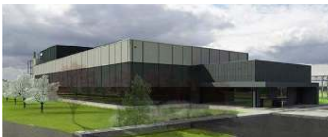
A €40m Pharmaceutical Facility in Dublin 22 at On-Site Stage
