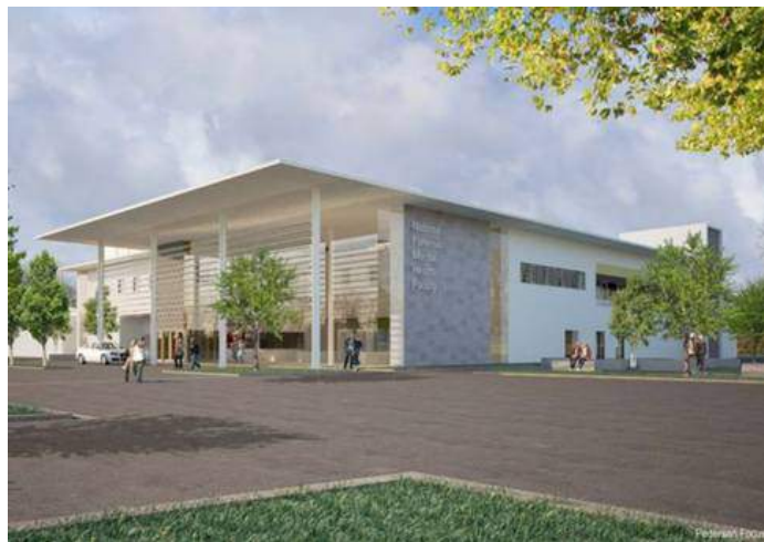
€125m National Forensic Mental Health Facility in Dublin at On-Site Stage
