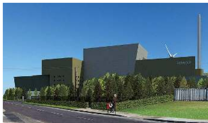
The €160m Waste to Energy Facility in Co. Cork.
