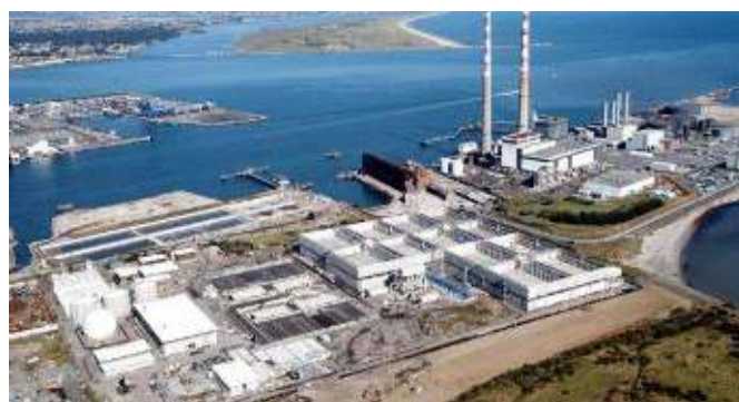
The €300m Water Treatment Plant Expansion in Ringsend, Dublin
