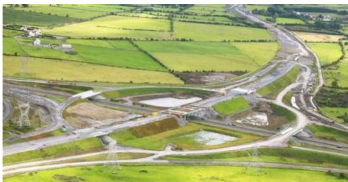
On-Site Gort to Tuam Motorway scheme
