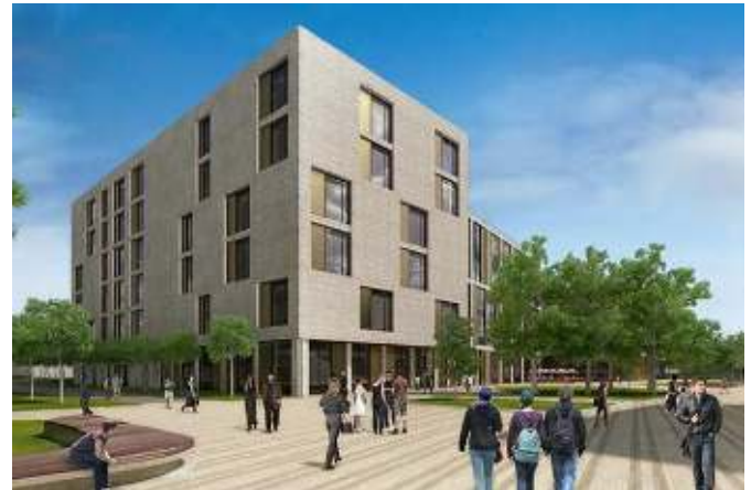
€70m East Quad Development at Grangegorman in Dublin at Plans Granted Stage
