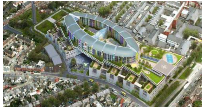
The €750m National Children's Hospital in Dublin at On-Site Stage
