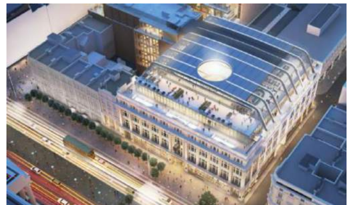
Clery's Store Redevelopment in Dublin City at Plans Submitted Stage
