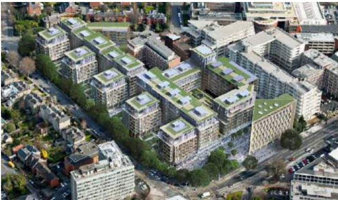
Residential Development in Ballsbridge, Dublin - On-Site Stage
