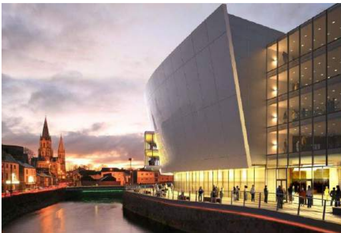
€53m Events and Convention Centre in Cork City at On-Site Stage
