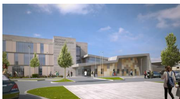
€40m National Rehabilitation Centre Project - Phase 1 at Tender Stage
