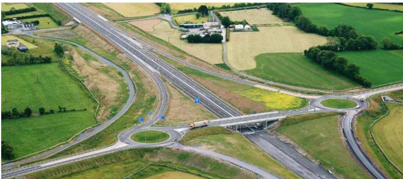
N11 Gorey to Enniscorthy PPP Road Scheme
